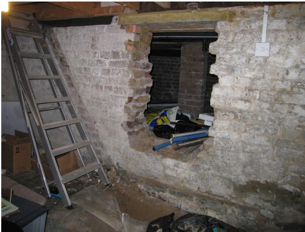
Photo 5 – basement to caretakers house
